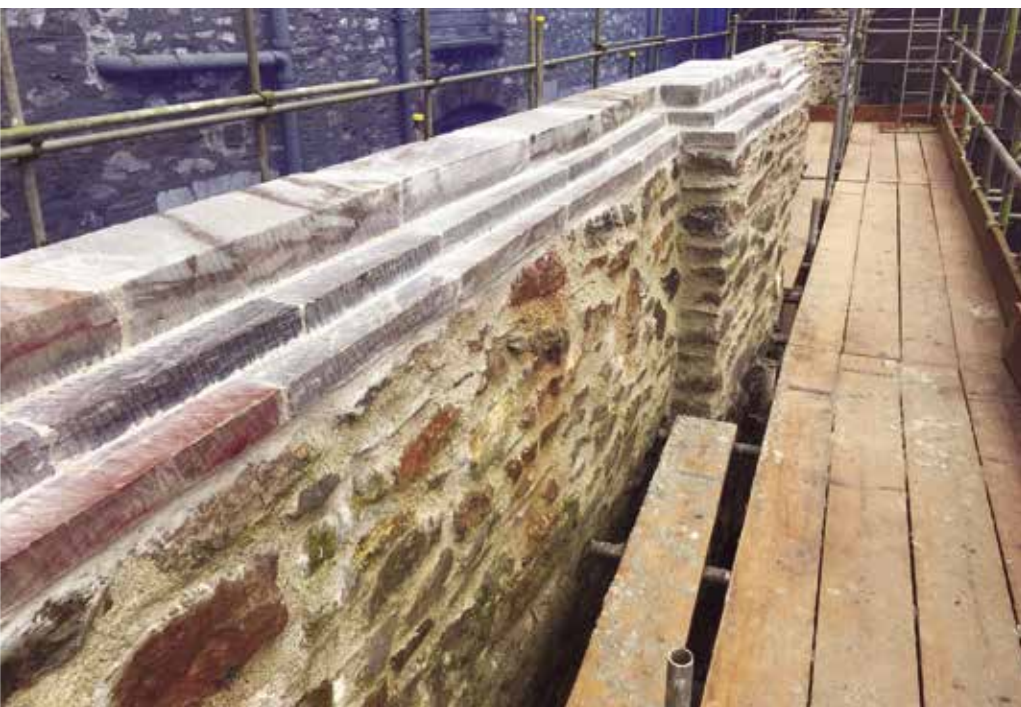
Left Repointing and new capping of the garden walls in Plymouth limestone
