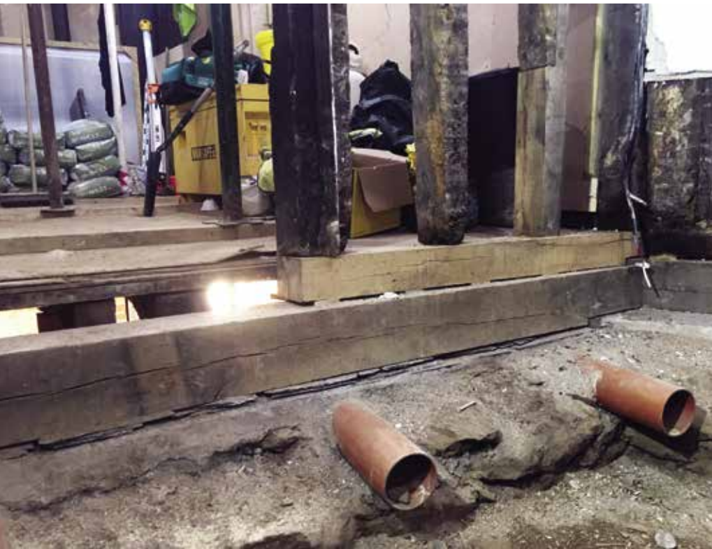
Above Oak sole plate repairs and ducts for radon protection on site
